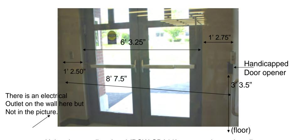
Using the two directional (PCW-SBA02) sensor, please describe how you would install it here (where and exactly how?). Are there multiple options?
